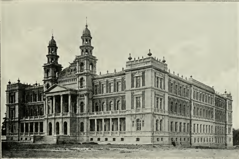
THE LAW COURTS AT PRETORIA. This building was finished just before the English occupied Pretoria (5 June 1900), but had never been used. The British turned it into a hospital. In a short time, this large building was full of sick and wounded.
